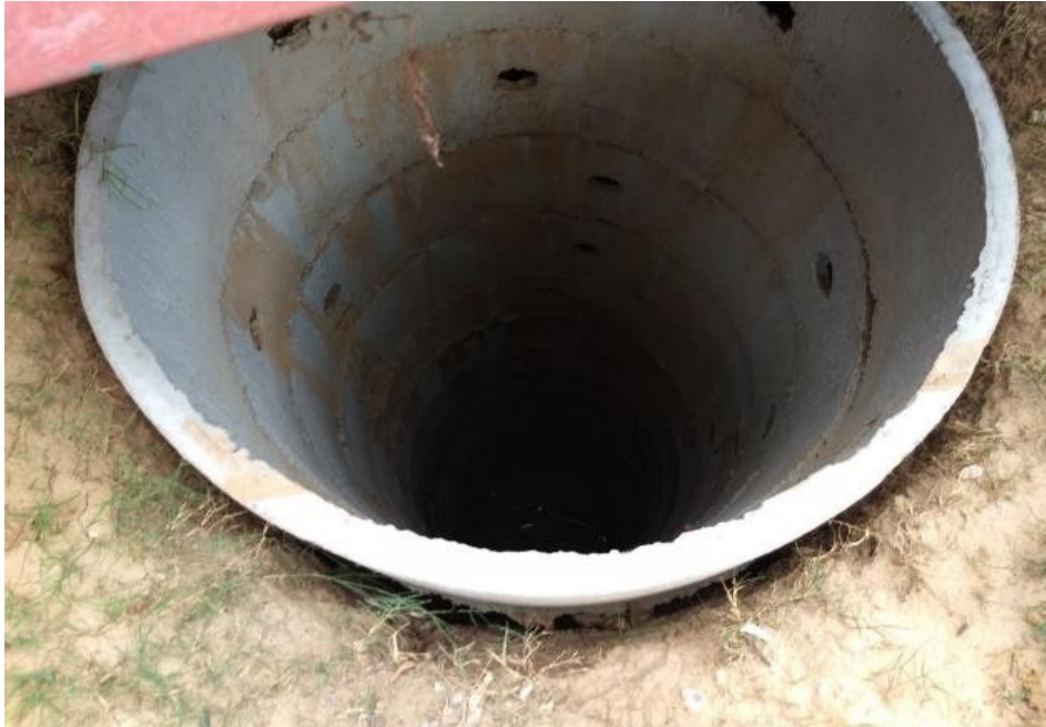
Rainwater Recharge Pit
