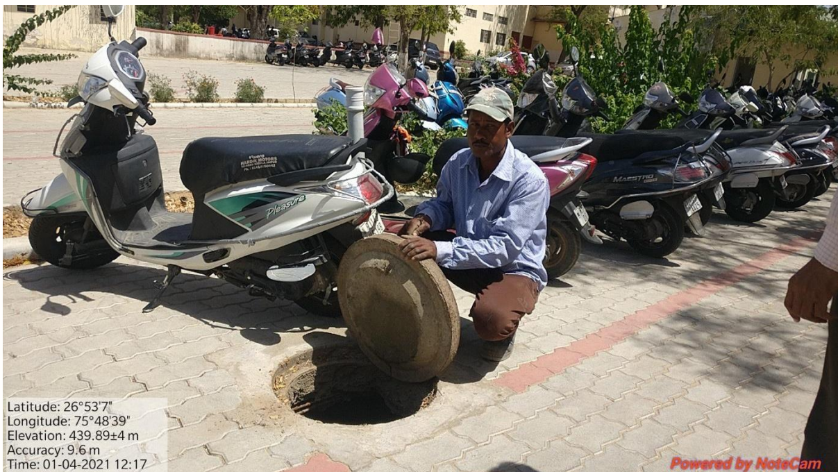
Rain water harvesting unit
